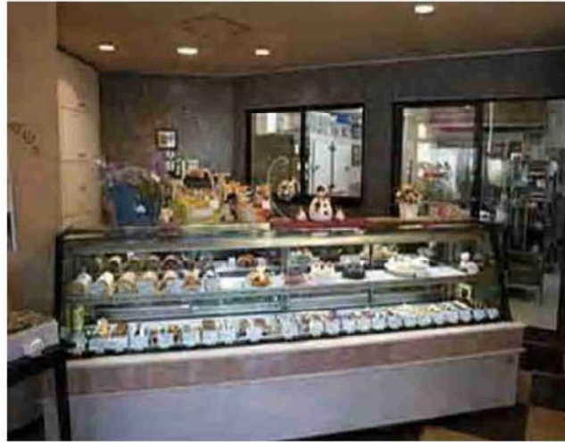
Photo 3 Showcase after dew condensation countermeasures taken
